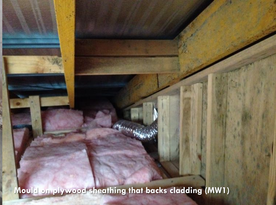
Sodden batts in contact with vapour impermeable wrap and metal cladding (no continuous cavity)
